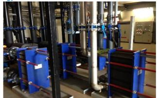
Fig. 3 Plate heat exchangers as part of an ATES system
