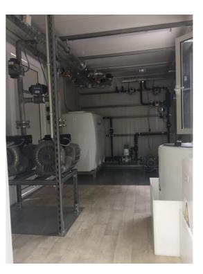
Figure 3. Images of the MBR used in NextGen project.
