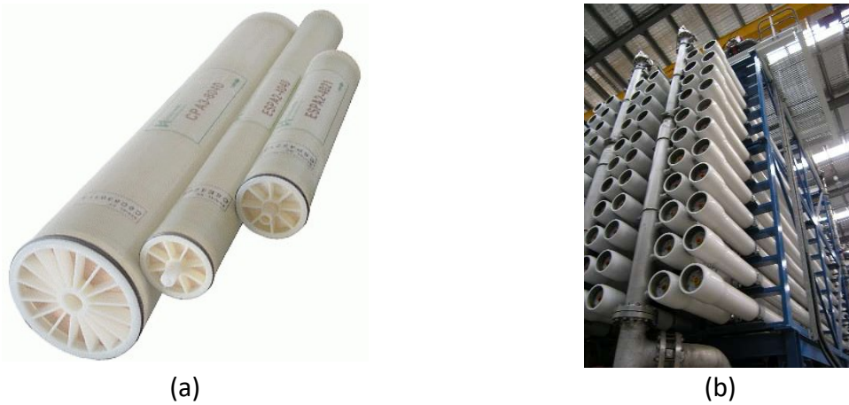
Fig. 4 RO membrane (a) elements and (b) pressure vessels.
