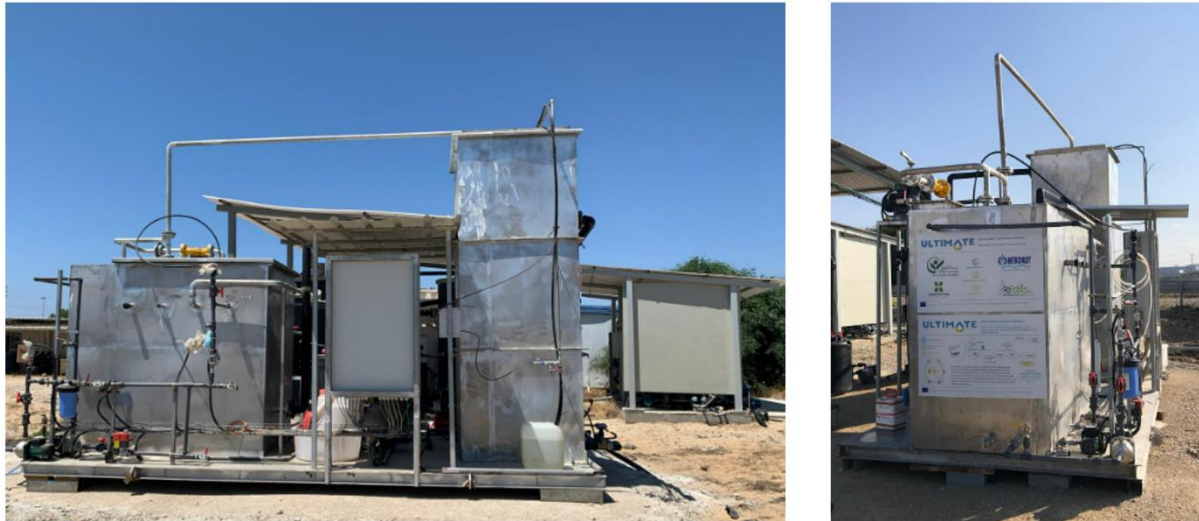
Fig. 4 Picture of the AAT combined with the AC/AnMBR at the wastewater treatment plant in Shafdan
