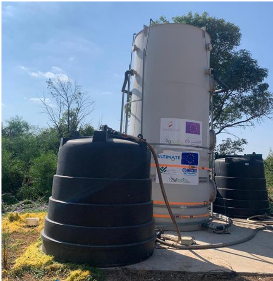
Fig. 3 Picture of the immobilised anaerobic high rate reactor at the wastewater treatment plant in Karmiel
