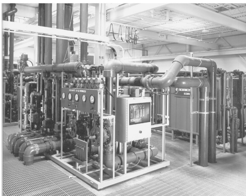
Fig. 11. Industrial size electrodialysis reversal (EDR) drinking water plant (photograph courtesy of Ionics Incorporated).
